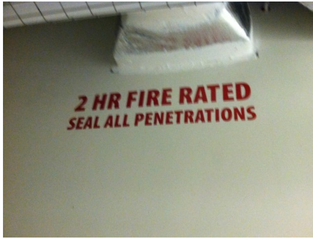
Photo 1 – Fire Wall Label Example #1
